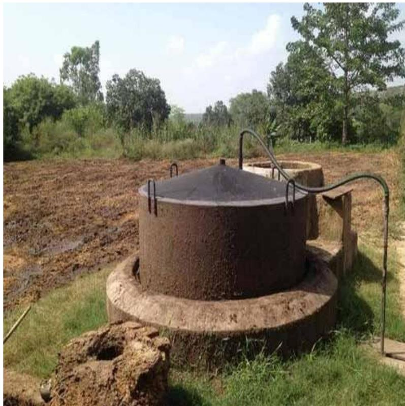
**Biogas Plant:** A biogas plant is the name often given to an anaerobic digester that treats waste or energy crops. Biogas can be produced using anaerobic digesters. A biogas plant consists of the following things:
