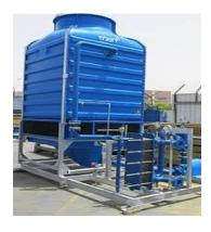
It's a device which cools the water by allowing it to fall through air flow which may be natural or forced so as to achieve evaporative cooling.
