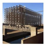
A condenser's function is to allow high pressure and temperature refrigerant vapor to condense and eject heat.
